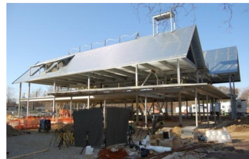
Actual picture of Structural System erected on schedule showing the accuracy of the 4D & 3D combination
