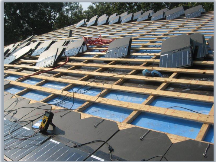
Figure 12 SUNSLATE installation
