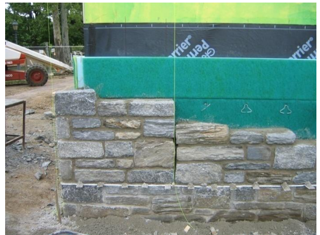
Figure 1 Existing Stone Veneer Construction
